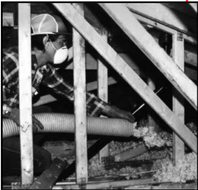
ThermaTech Attic Blowing Wool is granular insulation consisting of mineral fibers formed into nodules for installation by pneumatic machine.
